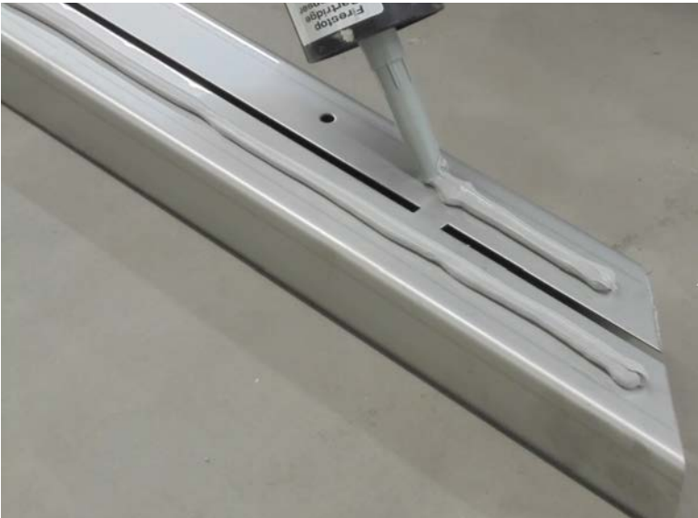
Apply silicone to the bottom side of the U-profile.
