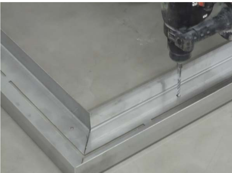
Dowel profiles tightly to the ground.
